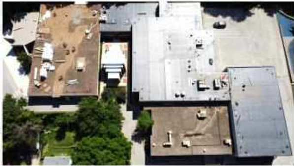
School roof, parish hall tile floor, and School gym partition wall
